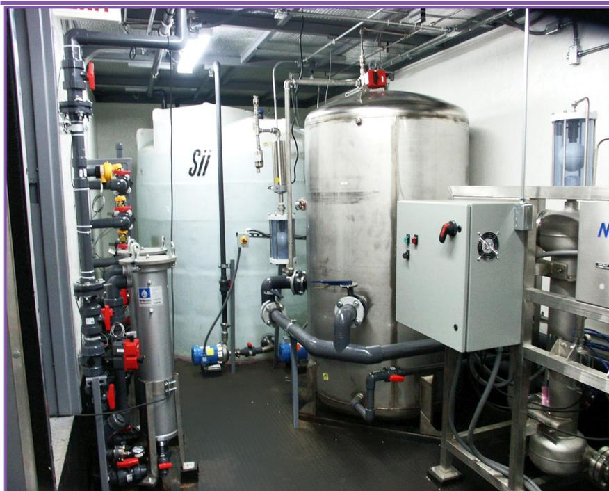
Figure 5. Advanced Oxidation process in Ohio<sup>10</sup>
