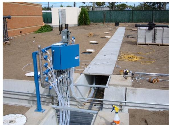
Figure 5: Ozone well field installation
